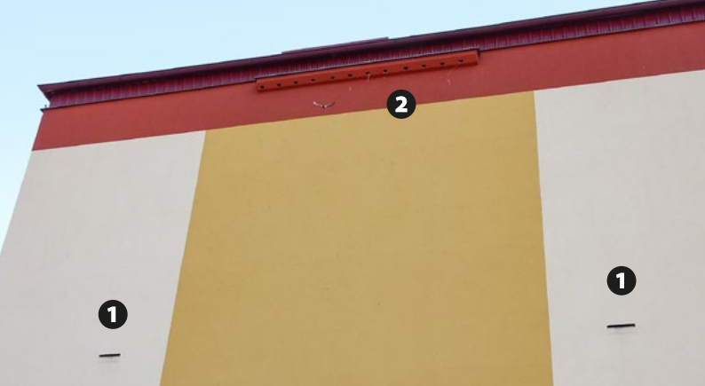
Preservation of nest sites and roosts using boxes: bat boxes hidden in the insulation layer (1), a multi-chamber nest box for colonially breeding swifts (2).
